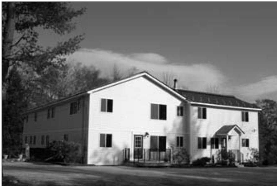
Saint Paul's House: now finished with new siding, windows, doors, roof, and entrances.
