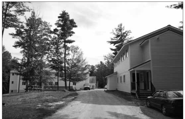
The new exteriors of all three Center buildings are now complete.
