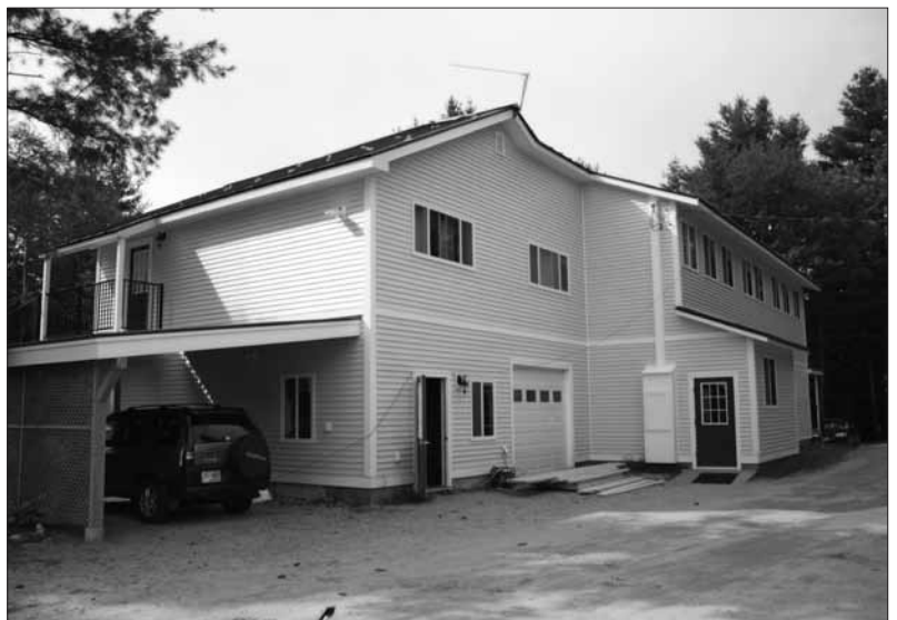
Saint Joseph's Hall with new siding, windows, and doors
