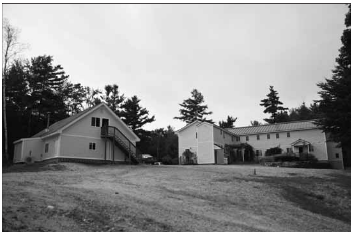
Saint Francis de Sales, to the left of Saint Paul's House, is newly sided.
